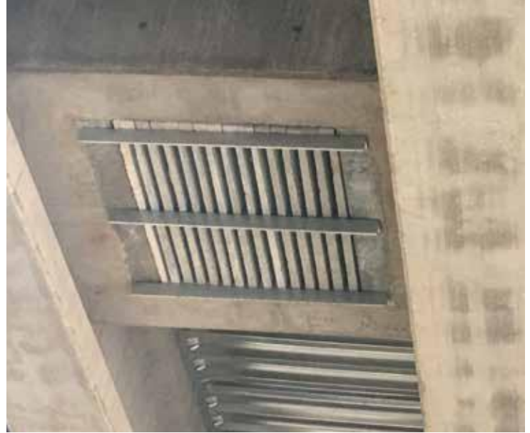
New bat boxes under the Ina bridge, Arizona Game and Fish Department
